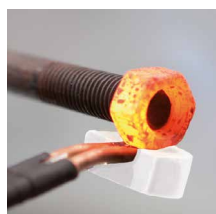
Releasing of rusted bolts
